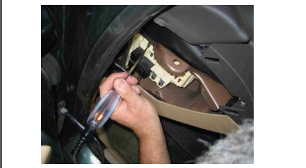
FIGURE 14-26 Testing a fuse with a test light. If the fuse is good, the test light should light on both sides (power side and load side) of the fuse.
