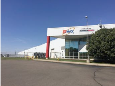
FIGURE 23–1 DMAX plant is located near I-75, and railroad access makes transport of materials and finished engines easy from Ohio plant.
